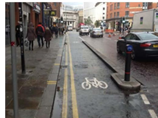
Photo 44: Oxford Street Back to Back Segregation Kerbing
