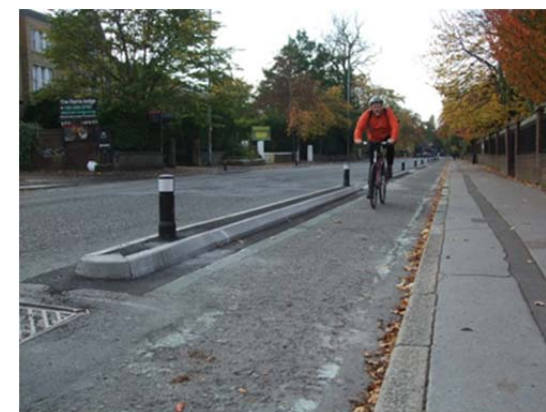
Photo 34: Northbound segregated cycle lane between Fallowfield and Withington
