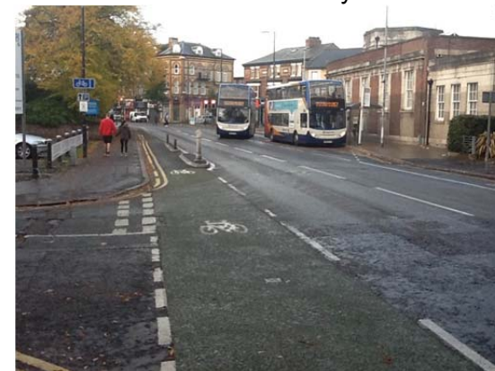
Photo 40: Bound green integrated into wearing course surfacing across side road entry Withington
