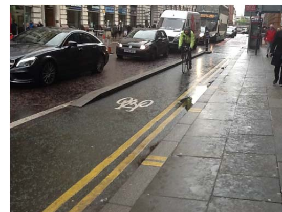
Photo 36: Photo showing back to back segregation on Oxford Road
