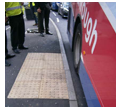
Photo 45: Photo showing lack of space between bus and kerb adjacent to island within Rusholme
