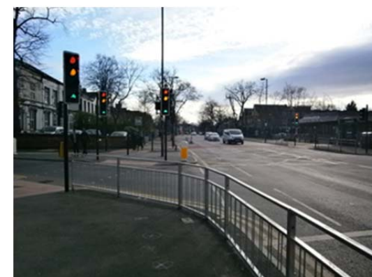
Photo 8: Wilmslow Road Fallowfield Egerton Road Junction looking southbound after construction showing early start signal for cyclists
