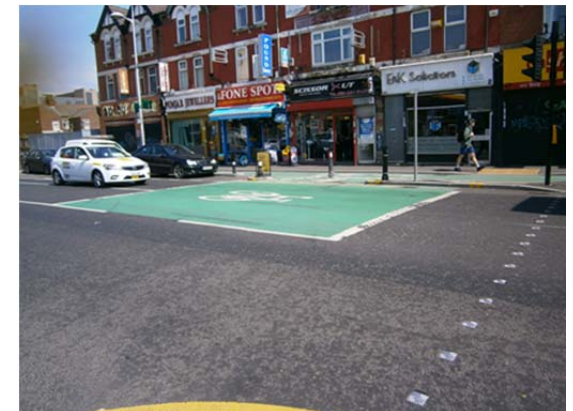
Photo 31: Surfacing colour tint applied to road wearing course in Rusholme
