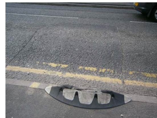
Photo 43: Damaged plastic light segregation orca in Fallowfield
