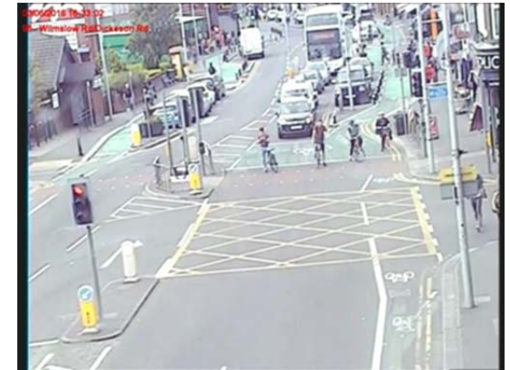
Photo 20: Camera 96 Looking Northbound across Dickenson Rd Junction showing cyclists putting the new 7.5m Advanced Stop Line to good use (irrespective of them all bar one being over the line)
