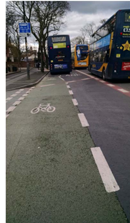
Photo 30: Bound green surfacing across side road on southbound approach to Fallowfield
