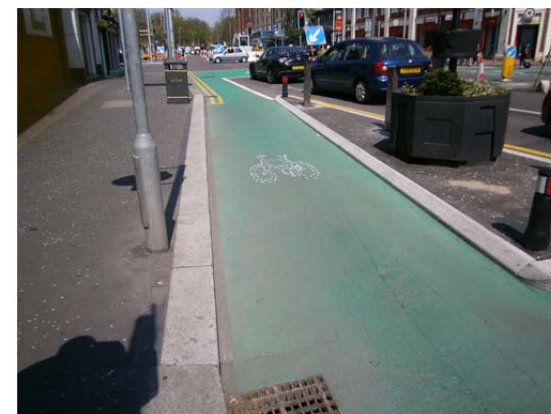
Photo 41: Green tint applied to surfacing in Rusholme
